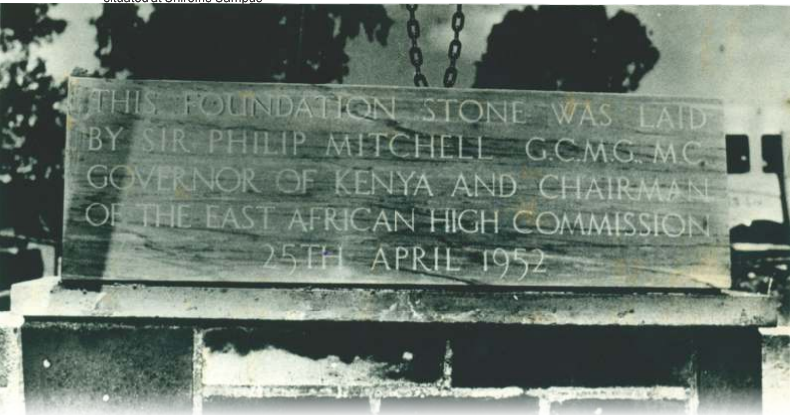
1952: Foundation stone of the Gandhi Wing Building at UoN Main Campus.
